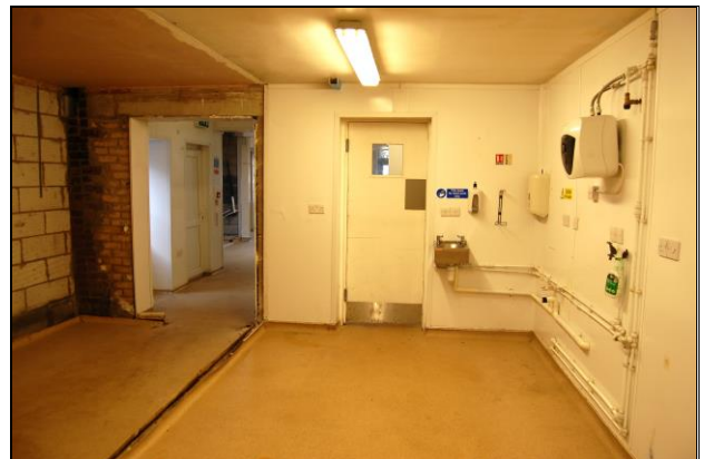
Store & Preparation Room
